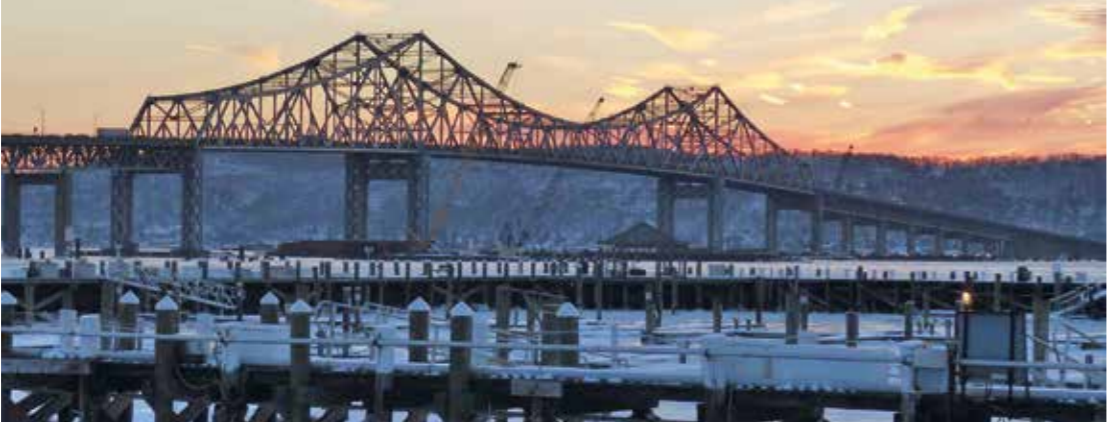
Observation de ponts (Tappan Zee Bridge USA)
